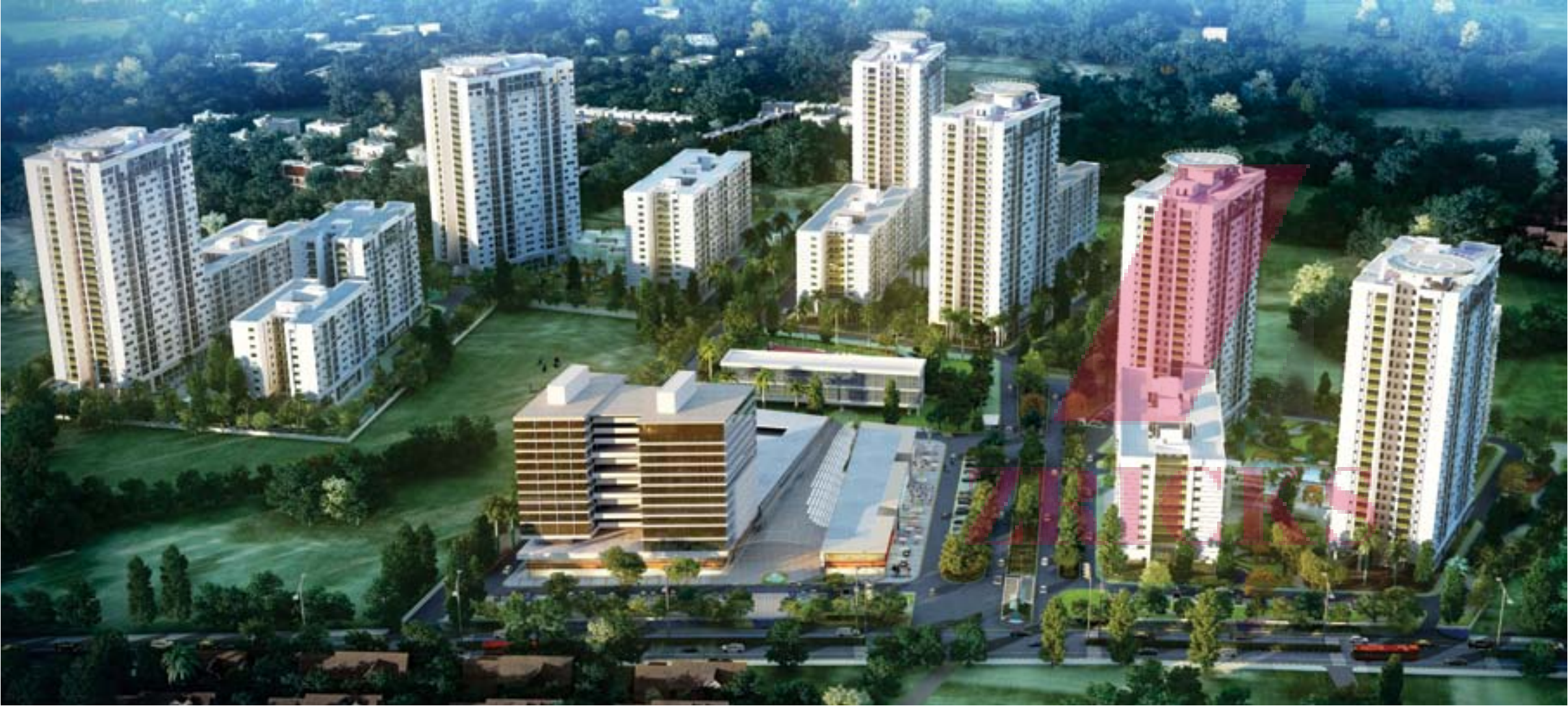
Aerial view of the Marq property
